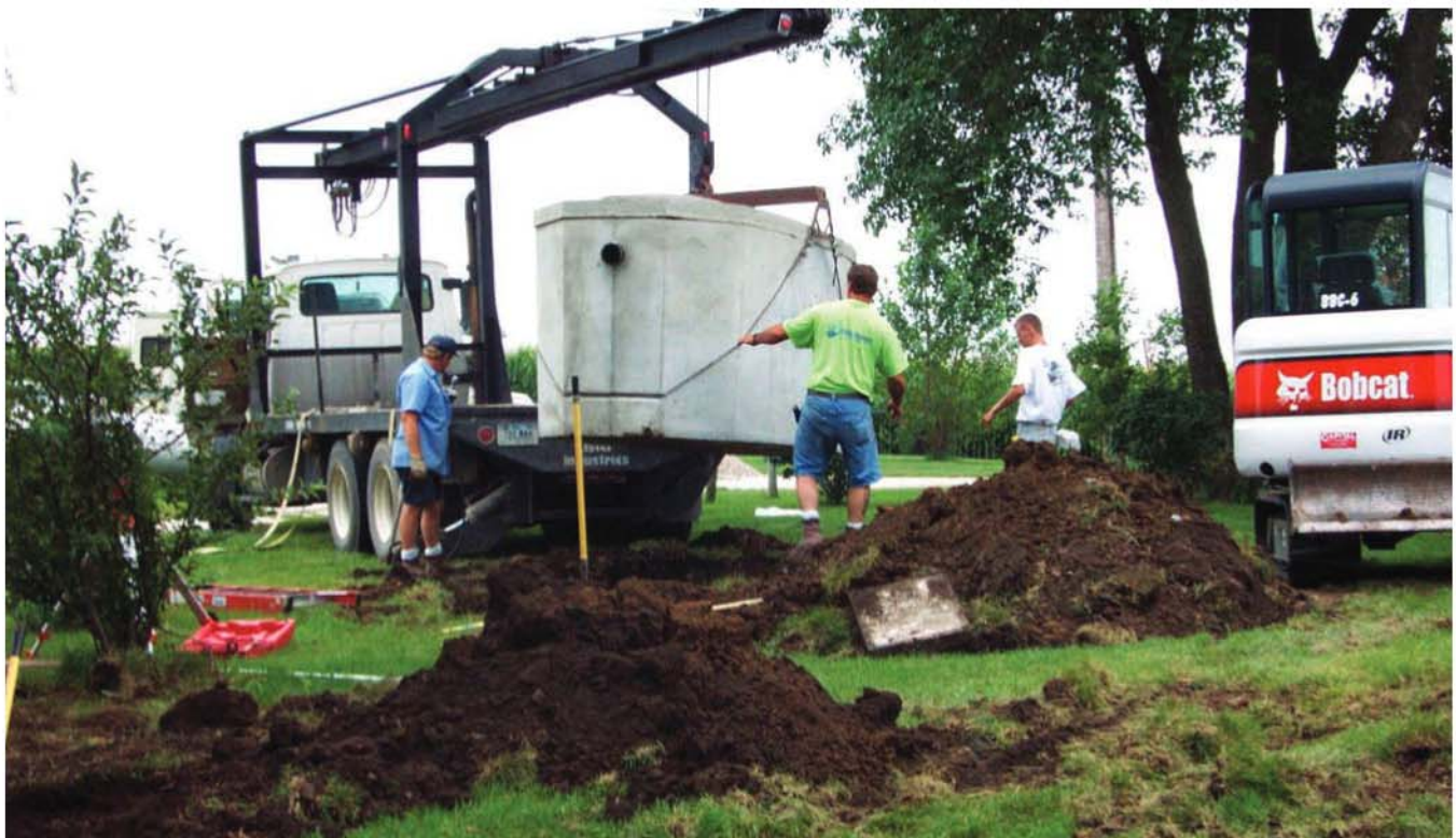
Installation of a new septic system.
